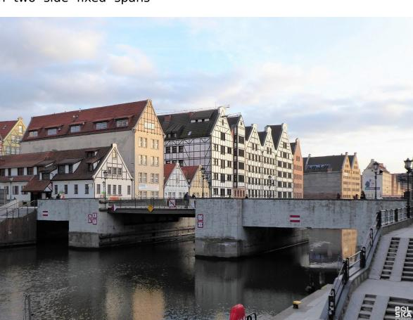
Over time, the lifting of the flaps was improved. After World War II, the central span of the Green Bridge was filled with concrete and immobilized without the possibility of launching, which stopped the movement of larger vessels deeper into the Motława River.
